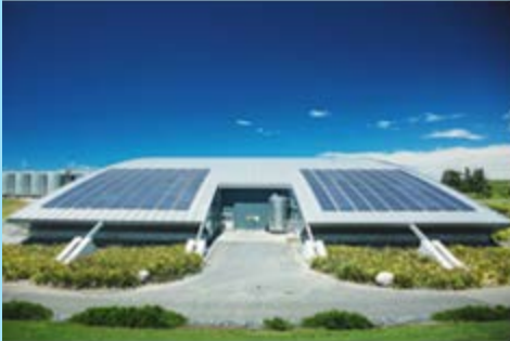
Solar Panel Installation
